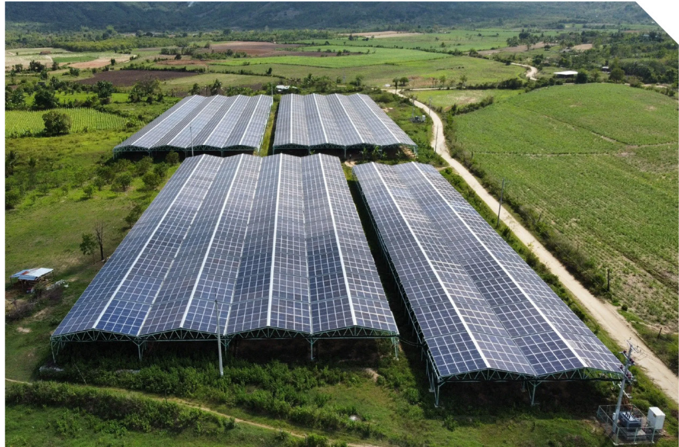
Photo: CAS Energy’s factory in Ninh Thuan province
