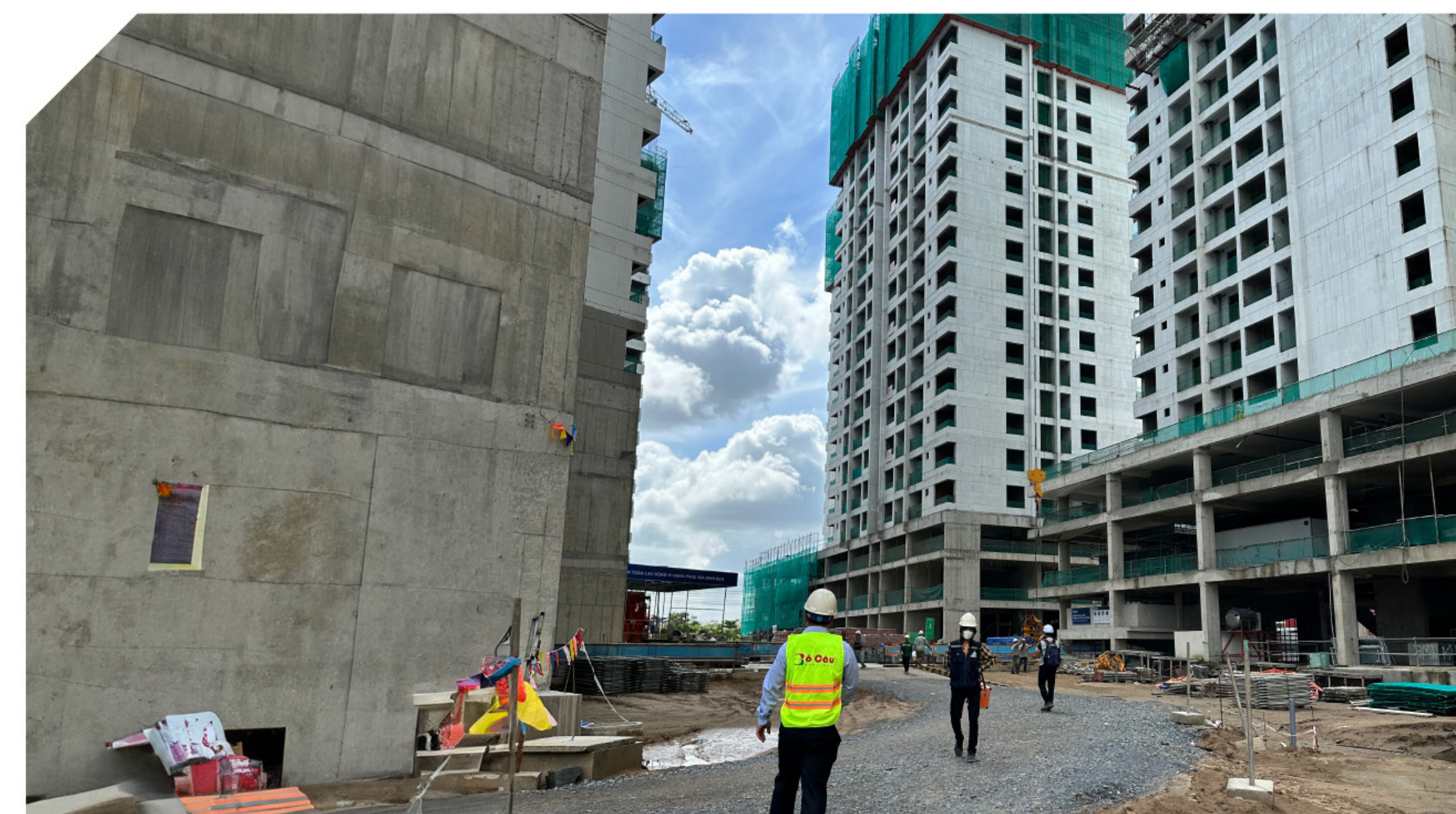
Photo: One of Bo Cau's telecom infrastructure construction sites in Vietnam
